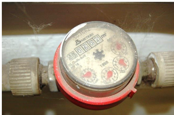
Obr. 69: VDM1 – Meranie spotreby SV pre ohrev TV
