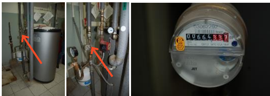
Obr. 4: VDM1 – Meranie spotreby SV pre ohrev TV
